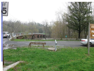
Duke Street Bridge over Swatara Creek.
